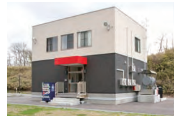
Equipped with seismic isolation, solar panels, rainwater tanks, and provisions needed for business continuity, the new building houses Myotoku's server computers.
