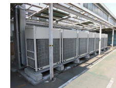
Updating HVAC equipment (Kofu Plant)
