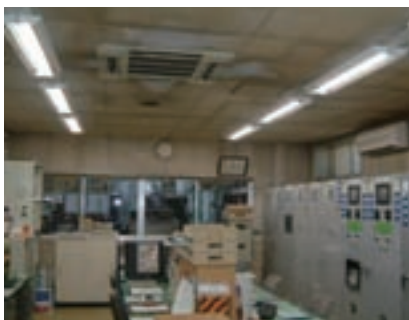
The Company's Mie Plant has adopted energy-saving lighting fixtures that employ high-frequency inverters.
